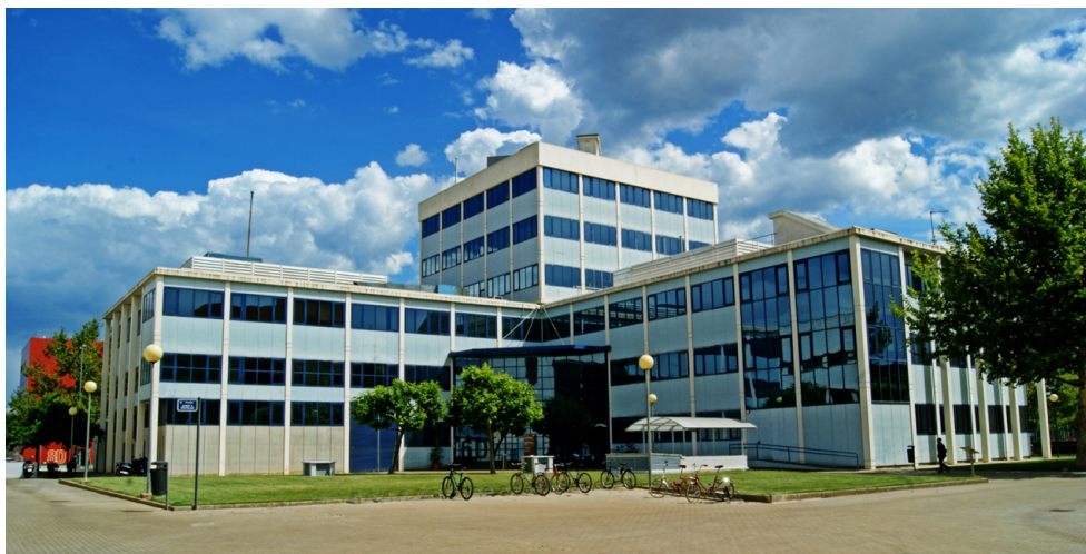
FIGURE 1: CMT Building at the UPV Campus.
