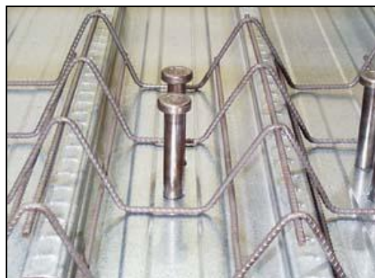
Picture 4.2.15: connectors that attach the plate to be forged Source: http://www.ferrosalonso.com
