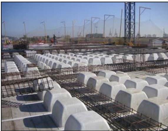
Picture 4.3.2.2: Installation of caissons and girders Source: http://www.celsa.com
