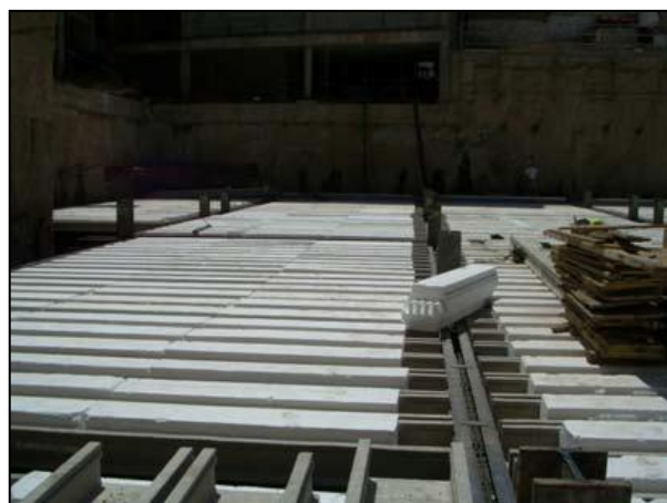
Picture 4.2.12: Mounting on steel beams pre-slab Source: Own picture
