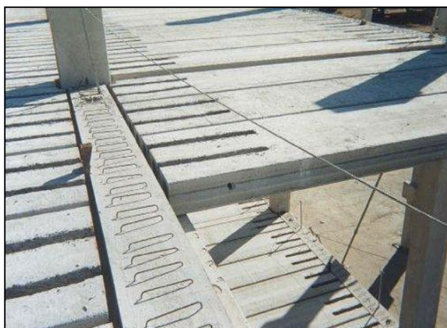
Picture 4.2.7: Union slab with precast beam Source: http://www.bison.co.uk/
