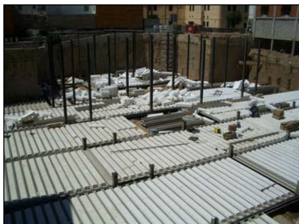
Picture 4.2.12: Mounting on steel beams pre-slab Source: Own picture
