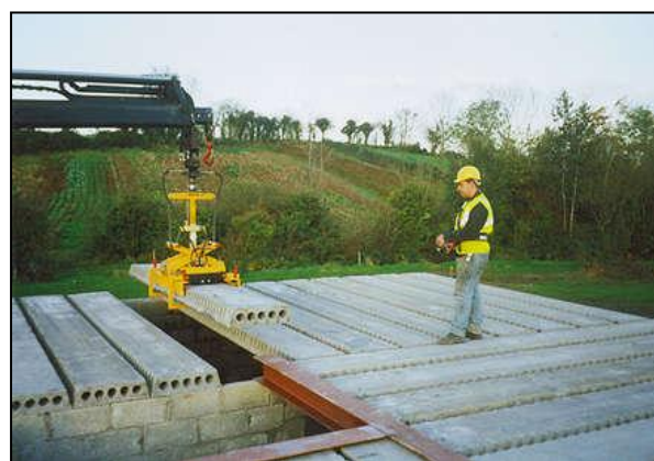
Picture 4.2.6: Positioning System alveolar slab
