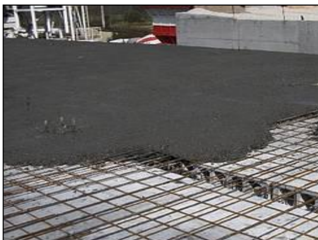
Picture 4.2.4: compression layer of corrugated steel mesh Source: http://esp.prefabricatspujol.com
