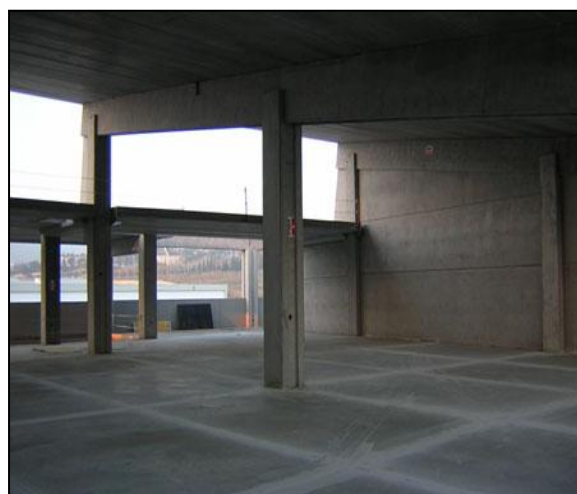
Picture 4.2.5: Parking and Warehouse made with hollow core slab. Source: http://esp.prefabricatspujol.com
