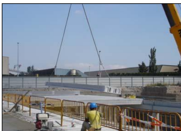
Picture 4.2.6: Positioning System alveolar slab
