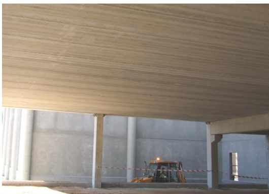
7.6. Placas alveolares forjado PF 30, PF 40, PF 50, Ref. Prevalesa
