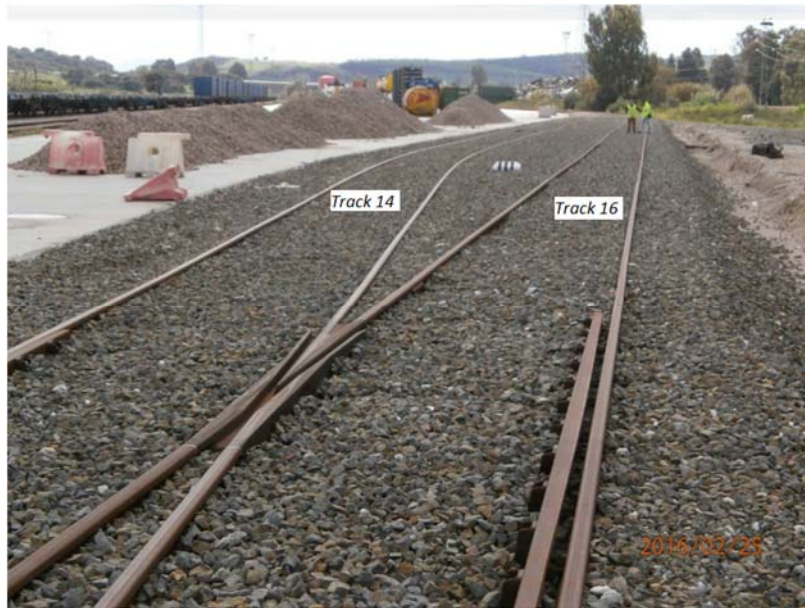
Figure 3. Tracks 14 (left) and 16 (right) after construction.
