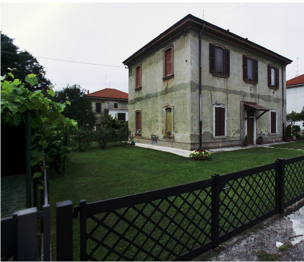
Figure 10. Worker's house in Crespi d'Adda, IT (Ian Spackman, 2007).
