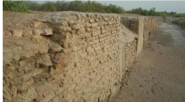
*Fig. 3 The brick are being attacked by the salted water from the back, of the inclining wall*
