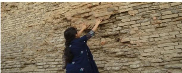
*Fig. 4 Showing salt penetration: into the pours of the bricks.*
