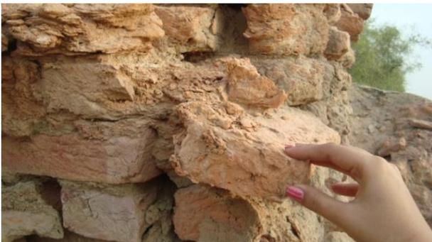
*Fig. 18 The wall brick deteriorating*
