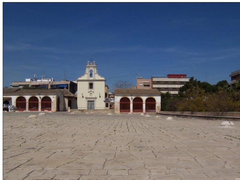
Figure 8. Valencian Silos Yard - General View (stock images)
