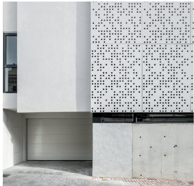
Figure 1. Facade, detail. 2017. ©Germán Cabo / Figura 1. Fachada, detalle. 2017. ©Germán Cabo.
