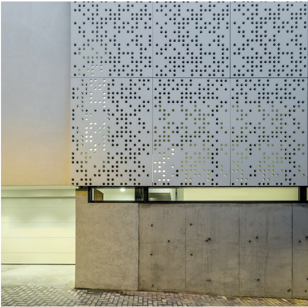
Figure 7. Facade (detail). 2017. ©Germán Cabo / Figura 7. Fachada (detalle). 2017. ©Germán Cabo.
