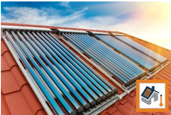
Figure 2.6: Evacuated Tube Collectors (ETC)
