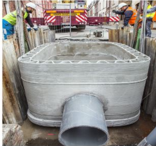
3D concrete printed storm drain
