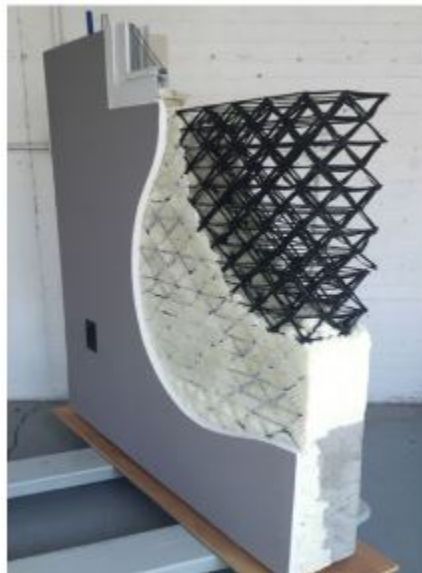
C-Fab Wall Partitions
