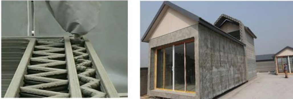
Internal reinforcement and 3D printed house
