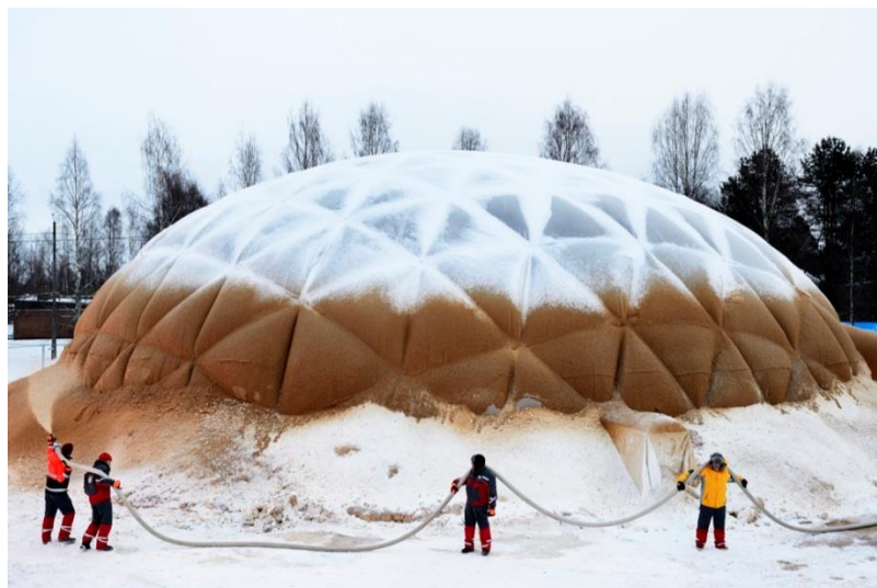
Figure 7.2: Pykete-reinforced ice dome built in Jukka, Finland, by the Eindhoven University of Technology. [Van14]
