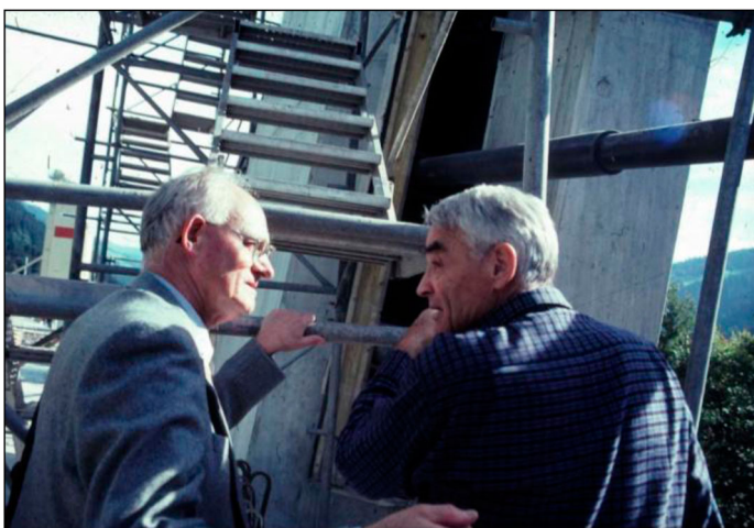
Fig. 3: David P. Billington (left) and Christian Menn (right) at the construction of the Sunniberg Bridge.
