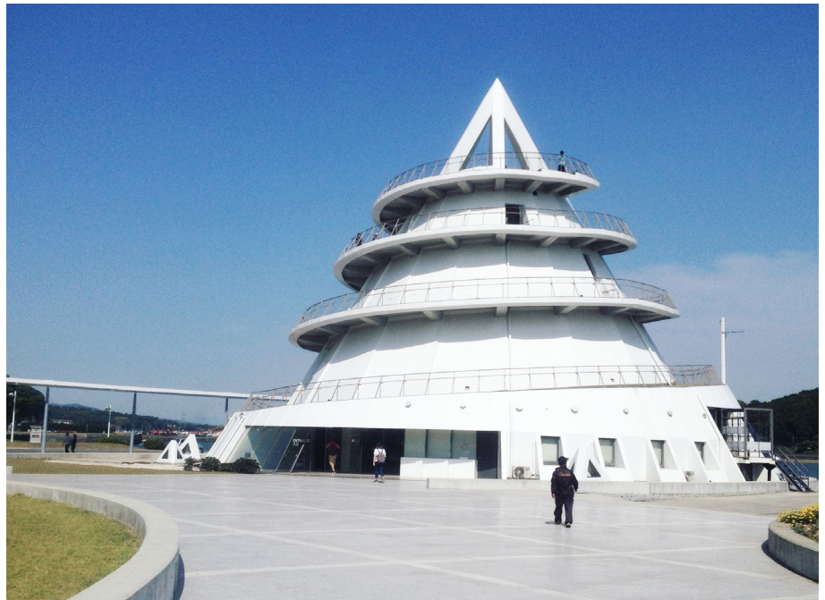
Misumi Ferry terminal. Shoei Yoh
