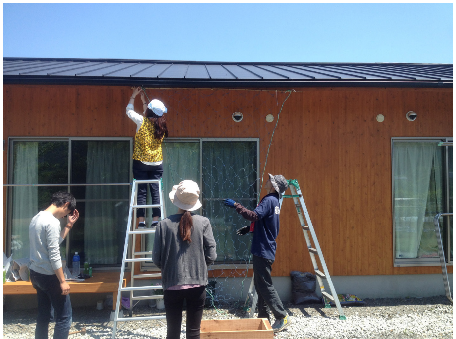
fitting the green solar shading
