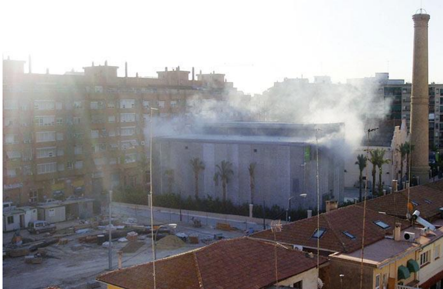
Figure 1. A photo of the substation during the explosion.
