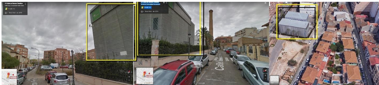
Figure 5. Vicinity of the substation.
