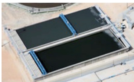
Figure 34 – (2) Pretreatment & primary settling (SUEZ, 2017)
