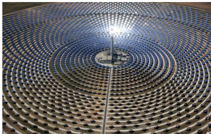
Figure 2-5. Gemasolar 20MW CSP plant, Spain.
