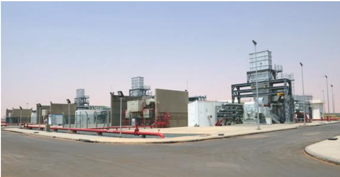
Figure 9 Saudi electricity company power plant in Sharoura.
