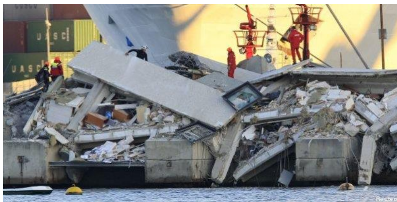
Figure 1-3 Effects of the impact of the cargo ship "Jolly Nero" against the mole of the Genova's dock.
