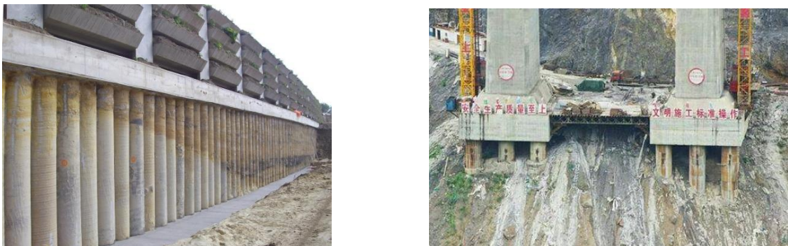
Figure 1-1 Examples of pile's foundations: the picture in the left side corresponds to a pile's wall placed in the city of Dresden (Germany); the picture in the right side corresponds to the pile's foundation of the bridge Zhou Jianhe (China).
