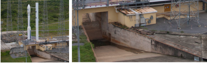
Figure 2.1: VEGA launch pad (left), and detail of the channel and the flame deflector (right).
