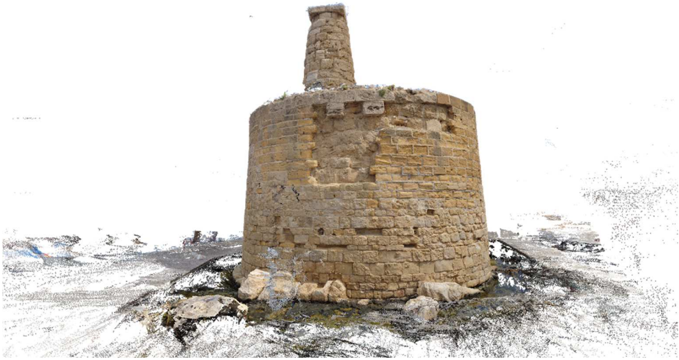
Fig. 9. A rendered west side view of the 3D model, the added stone layer of the modern restoration is clearly visible (Griffo, 2018).
