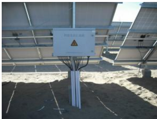
Figure 33: Solar string combiner boxes (Source: https://images.app.goo.gl/v4DHYSZ9Y4CziM8g6 )
