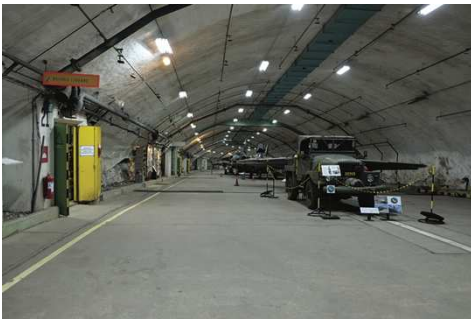
Fig. 1. The entrance gallery of Aerozeum, Gothenburg, one of the museums supported by the Swedish Military Heritage network (Sveriges militärhistoriska arv). It was a secret underground mountain base in the area next to Gothenburg. With an area of 22000 m 2 , today is a combination of museum, hands-on centre and conference facility. The development of the site started with the interest of the former general, which now is still part of the organisation, to keep objects from the military function and display the history of the air defence in Sweden. (Author, August 2019).
