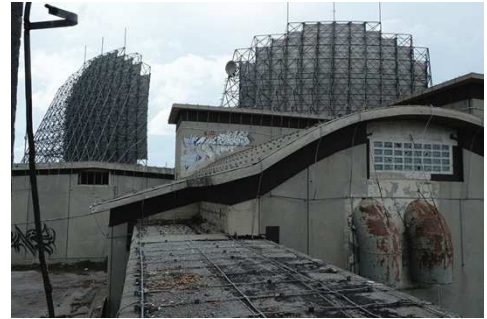
Fig. 4. Abandoned site of Dosso dei Galli, Brescia. (Author, July 2019).
