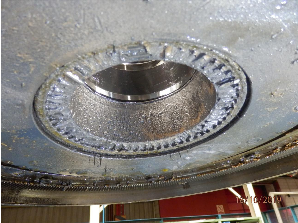
Figure 6: Damage of the piston.
