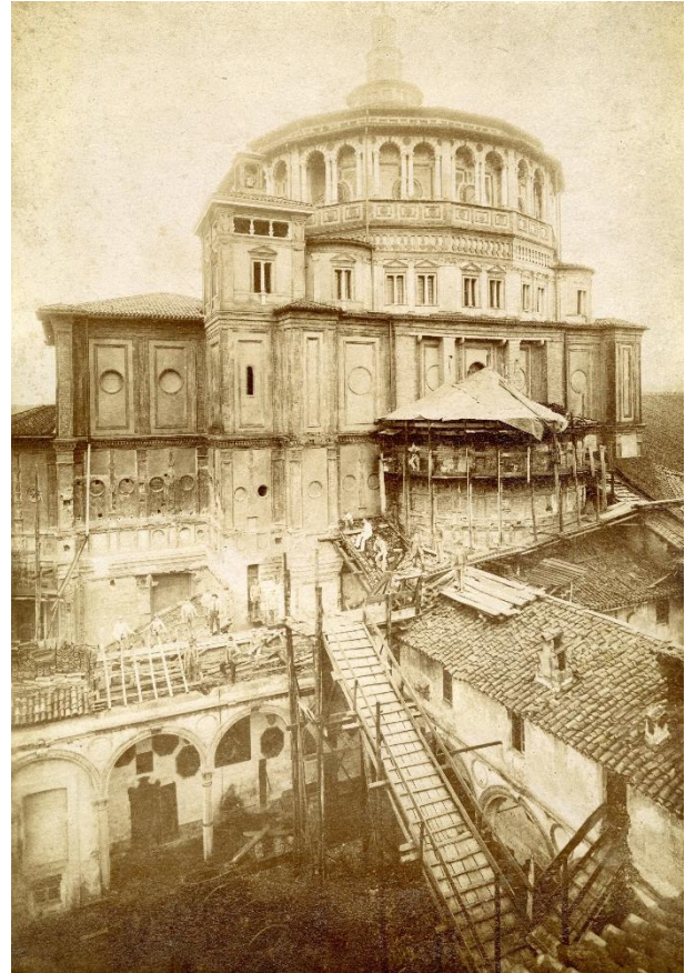
Figure 27: Period picture showing the roof of the Small Sacristy.
