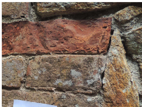
Fig. 15. Bricks of the internal jambs of the tunnel (Fratini).
