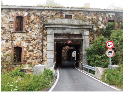
Fig. 4. The access to the tunnel (Fratini).
