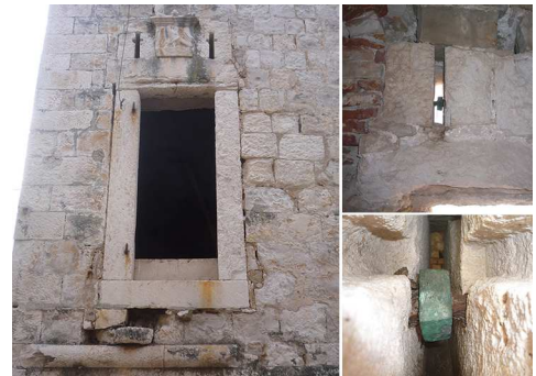
Fig. 10. Entrance on the first floor with the drawbridge lifting system remains (authors, 2019).
