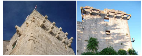
Fig. 16. (left) Machicolation corbels of the Aquila tower and (right) the Cerineo castle. 4
