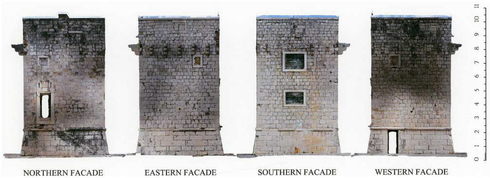
Fig. 4. Architectural survey of the Aquila tower facades obtained by a 3D laser scanner (Geographica d.o.o., 2018).
