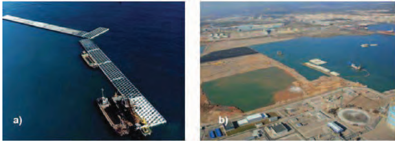
Figure 3: Conventional use of reflective caissons at Sagunto Port
