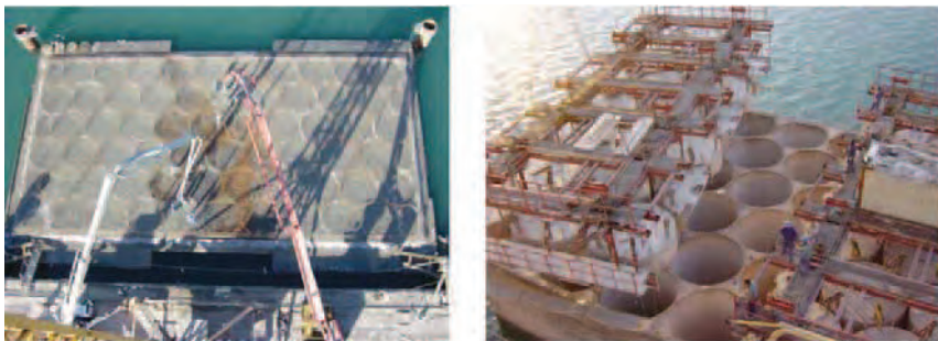
Figure 2: Floating dock and caisson fabrication in CYES installation
