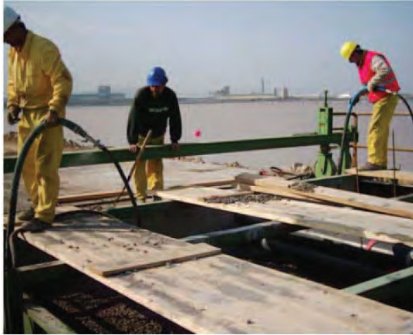
Figure 11.- Superstructure execution over quay wall caisson
