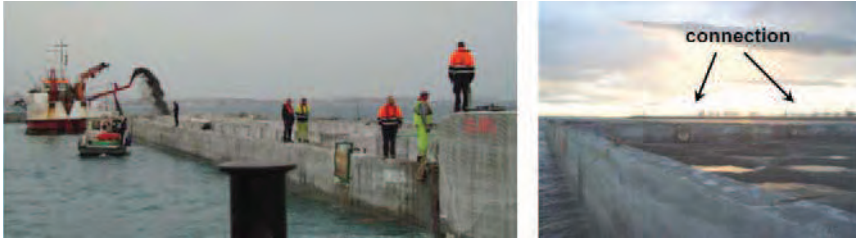
Figure 19: Caisson cells sand filling in Valencia Port.
