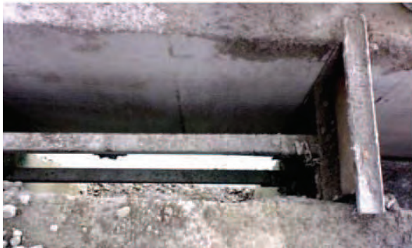
Figure 9.- Sealed pieces and cover protection for towing in manufacturing caisson process
