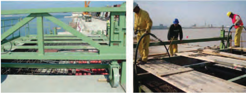
Figure 20: Superstructure execution over quay wall caisson
