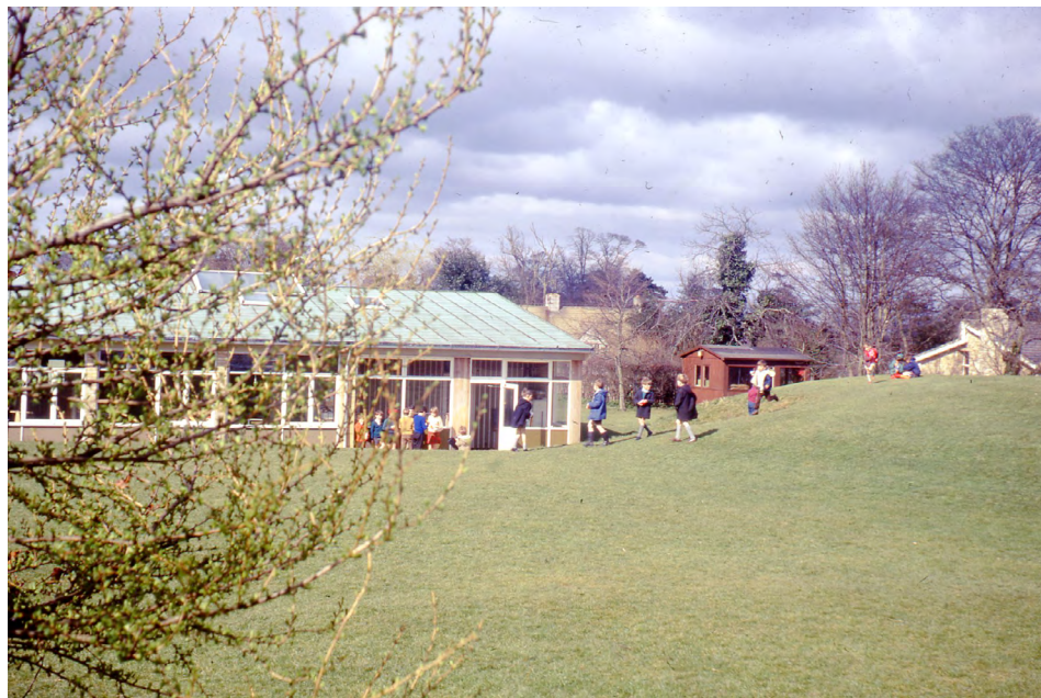
Exterior from field 5/4/73
