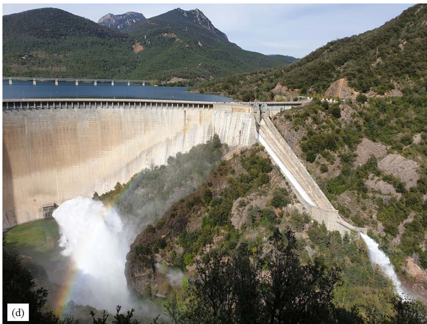
Figure 1. Discharge in large-dam spillways (courtesy of Dr. Gómez de Membrillera and Carlos Barbero): (a) Aguilar dam (Palencia, Spain), (b) Camporredondo dam (Palencia, Spain), (c) Brezina dam (El Bayadh, Algeria), (d) la Baells dam (Barcelona, Spain).
