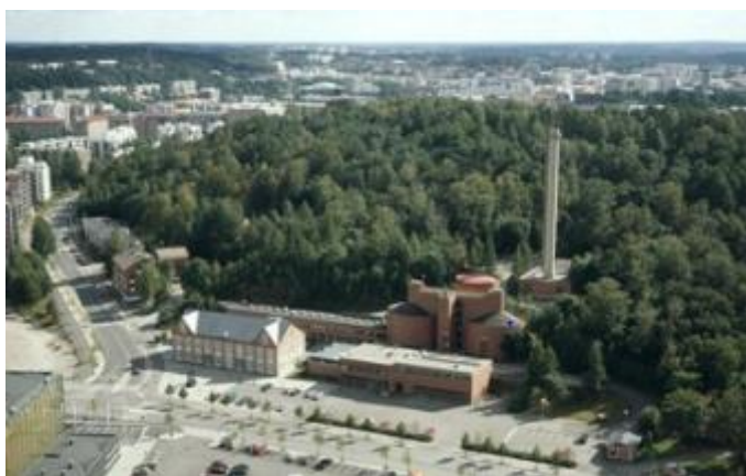
Image 1. Kariniemi wastewater treatment plant (Palmer 2016)
