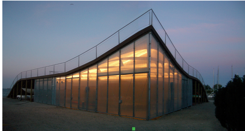
Maritime Youth House, Copenhagen_Bjarke Ingels Group y JDS architects
