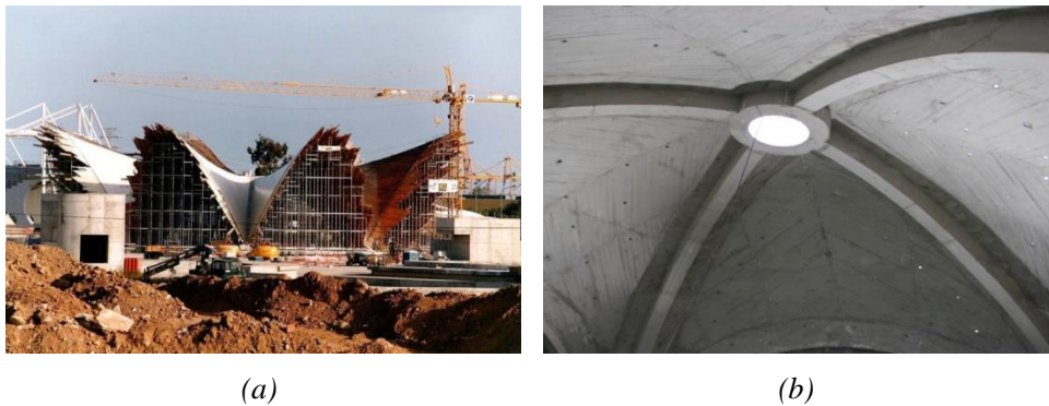
Figure 1-1: SFRC shell roof of the Oceanographic Park in Valencia, Spain [1] (a) and the PFRC vaults of the Cathedral de San Cristobal de la Laguna, Spain (b) [2].
