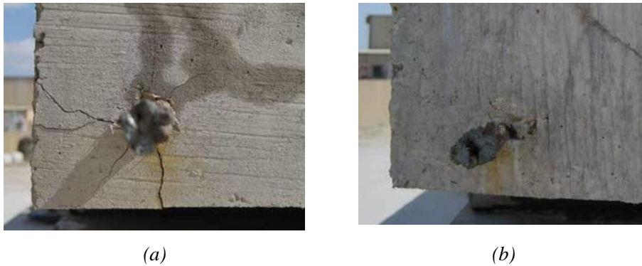
Figure 2-40: Prestressing strands at the end of specimens [190] ( a/d=2.73 ) at failure for the PC (a) and SFRC (b) slabs
