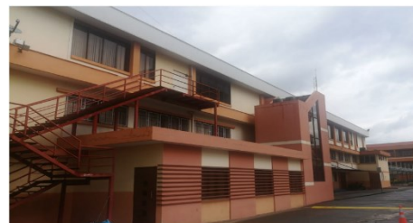
d) Data center
