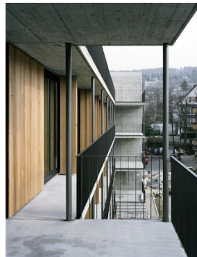
GRET LOEWENSBERG. HINTERBERGSTRASSE HOUSING BUILDING. ZÜRICH
