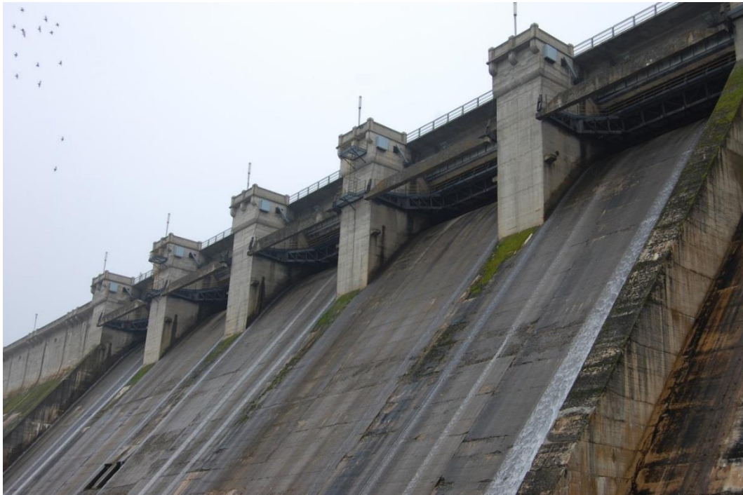
Figure 4-3. View of the Santa Teresa spillway from downstream.
