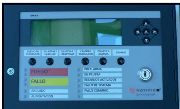
**Figura 3: Panel repetidor**
