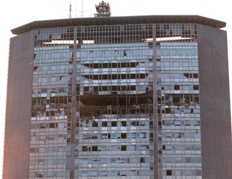
Figure 5.11: The building after the impact. Source: https://milano.fanpage.it [26].
