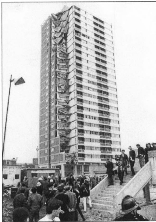
Figure 1.1: The Tower after the collapse of the angle. Source: Ronan Point Apartment Tower Collapse and its Effect on Building Codes [31].
