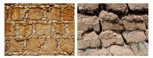
Figure 5. Cut earthen blocks: a) Marl; b) Sod (Authors).
