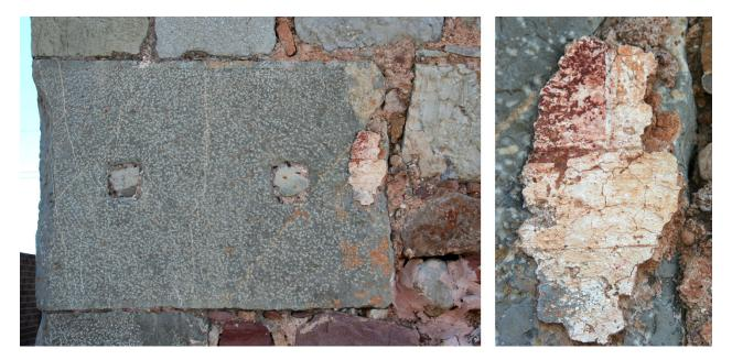
Fig. 14. Remains of the cladding on one of the corner ashlars, on the north flank. The incisions in the final layer that delimit the colour planes and the remains of reddish pigments and ashes can be clearly seen. It is not the only sample that remains on the battered façade. On the other hand, this corner ashlar seems reused, perhaps from a Roman construction. (Authors 2013).
