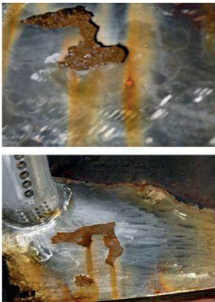
Figure 13: Detail of degradation with suction and turbine aeration pipes due to cavitations. (Source Endesa Generación-Enel Green Power).
