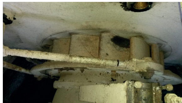
Figure 2: Distributor and turbine blades. (Source Endesa Generación-Enel Green Power).
