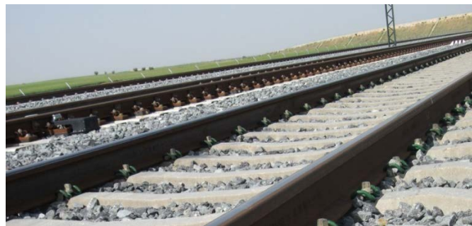
Fig. 3. Ballast track superstructure in Spain.
