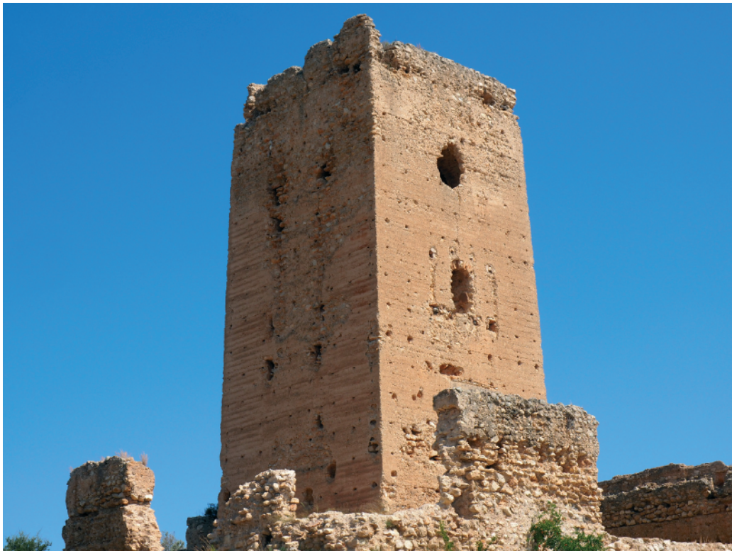
Figure 16. Tower of the castle of Aledua, Llombai. Source: authors
