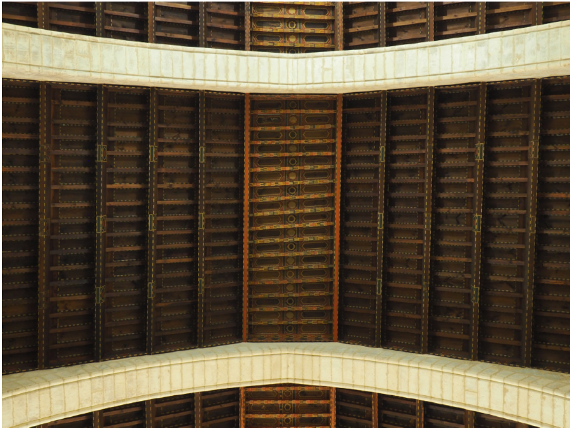
Figure 13. Roofing church San Pedro, Xàtiva. Source: authors
