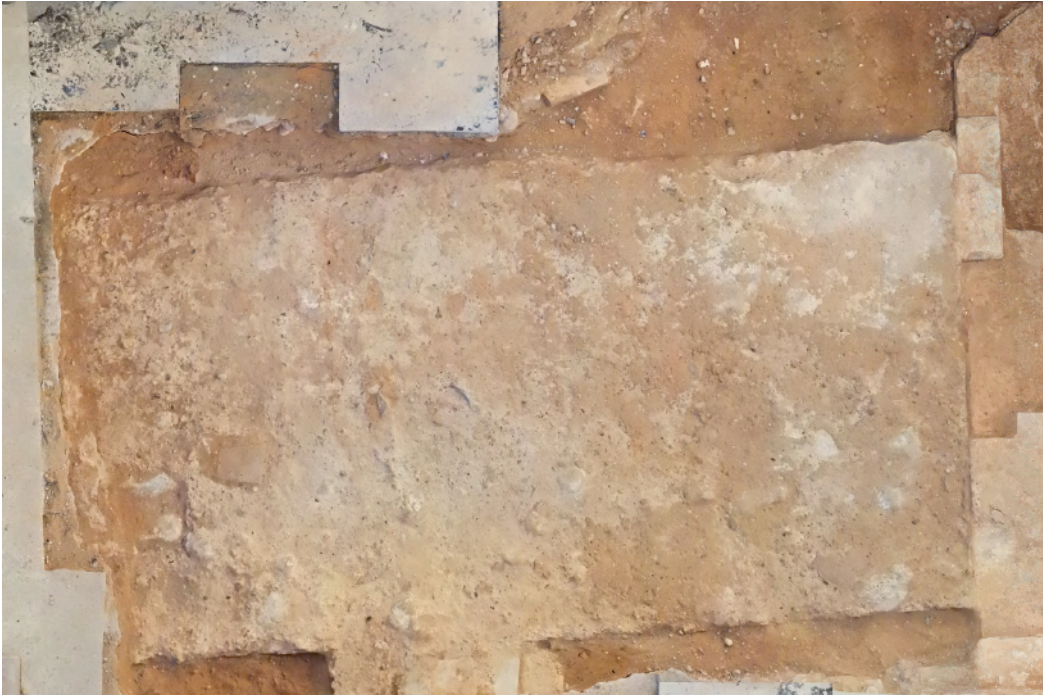
Figure 17. Lateral wall of the 13 th century bell tower, the bottom of which used the buttress of the diaphragm arch to close the structure (exploration 1). Source: authors
