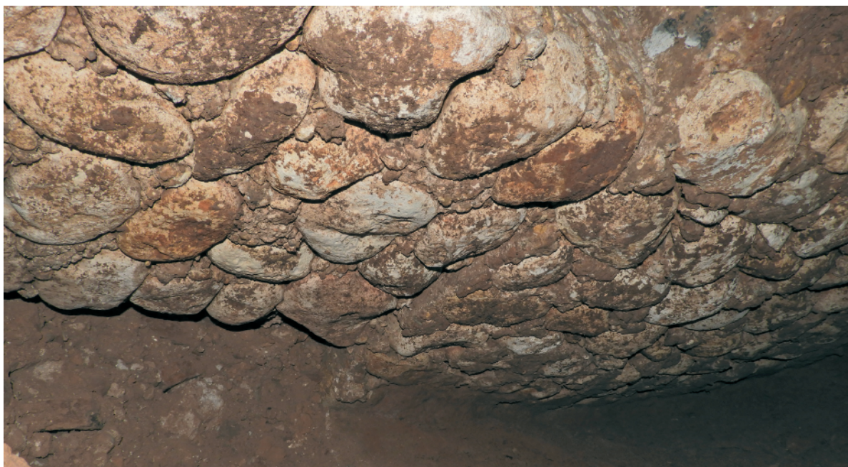
Figure 12. Regularization layer (top view, exploration 1). Source: authors
