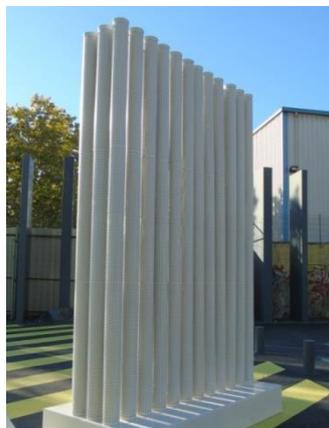
Figure 6: Sonic Crystal Acoustic Screen.
