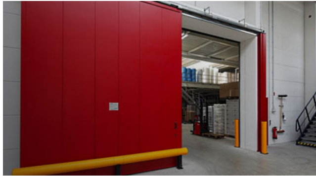
Figure 5.19 Industrial sliding fire resistance steel door. Picture extracted from Samson doors official website [6]
