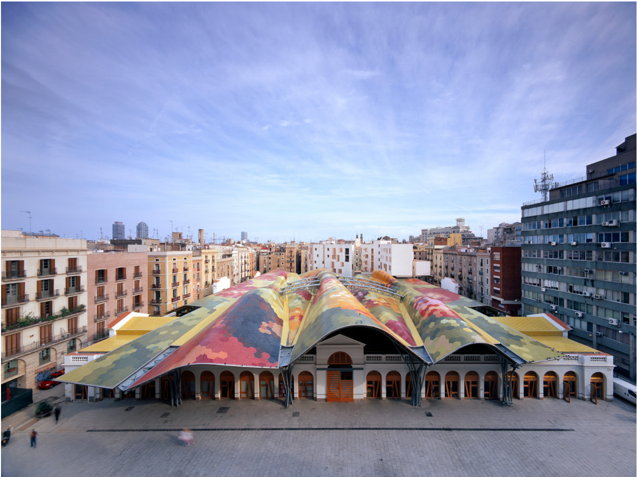
Figure 1 | Santa Caterina Market. Barcelona, Spain 2005. Photo: Roland Halbe.
