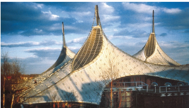
Figure 14. High point with a cable loop in a cable net. German Pavilion. Montreal Expo 1967. ©Atelier Frei Otto + Partner.
