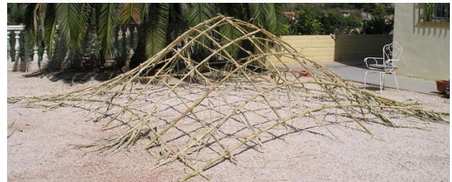
Figure 24. Self-built reed gridshell. ©Author's photograph.
