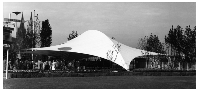
Figure 10. Arch-supported entrance canopy. Federal Garden Show. Cologne, 1957. ©Atelier Frei Otto + Partner.
