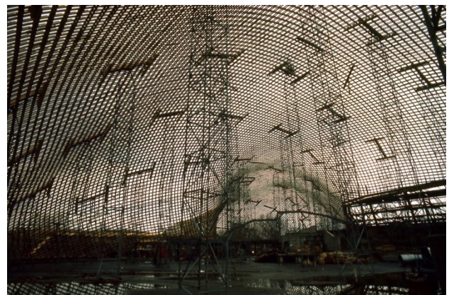
Figure 22. Building process of Mannheim Multihalle gridshell. ©Atelier Frei Otto + Partner.
