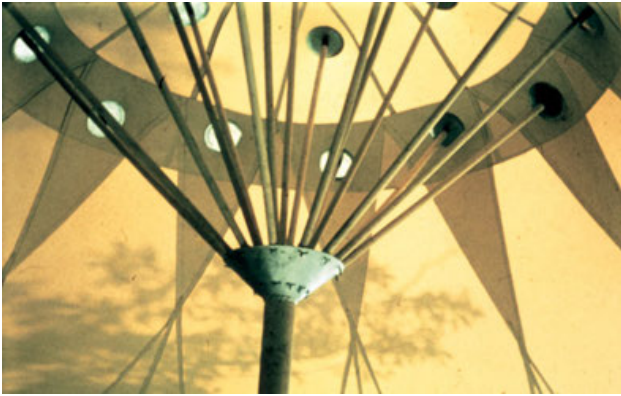
Figure 12. Mast tip split in a bundle of rods. Federal Garden Show. Cologne, 1957. ©Atelier Frei Otto + Partner.
