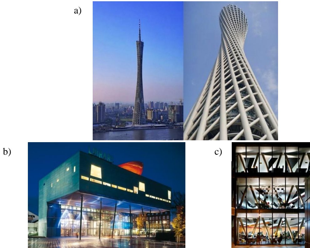
Fig. 3. Examples of buildings using CFST columns: a) Canton Tower (Guangzhou, China); b) Peckham library (London, UK); c) Marguerite Yourcenar Media Library (Paris, France) [16].
