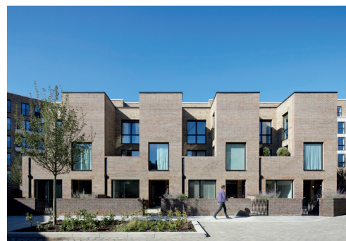
Figura 46: Vivienda, Chobham Manor
