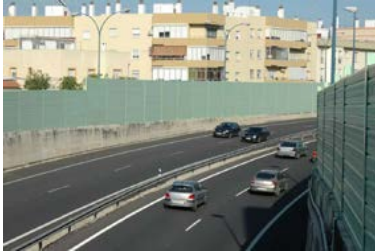
Figure 10: Acoustic barriers in between residential areas of the city of San Fernando (Spain).
