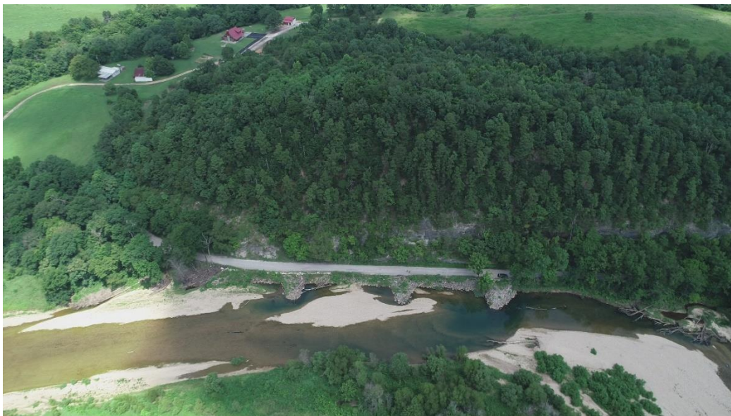
Figure 52 - Reach 2, 2021 drone pictures showing the existing structures protecting the road
