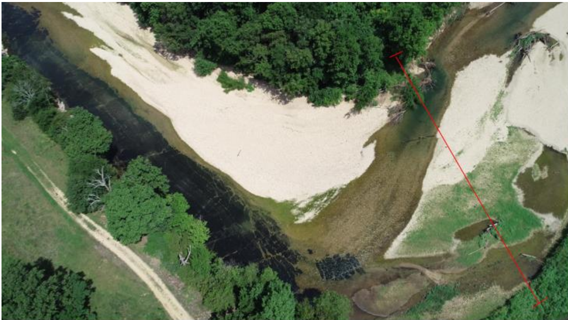
Figure 45 – Cross-section 8 in red showing the trees blocking the flow of water.
